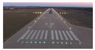
Lights across runways and taxiways require constant verification & maintenance. We have developed a reliable solution that quickly detects malfunctions such as lights off or with incorrect colour.
