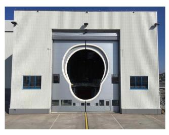
productivity. Such an arrangement also means that MRO operations can be undertaken on larger Code E and F aircraft in hangars that would otherwise be too small.
