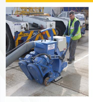
This method uses highly abrasive particles to force marking material from the attached surface. This technique is effective at removing marking material from the surface, but it is very slow, more expensive and commonly causes potential Foreign Object Debris (FOD) hazard for aircraft.
